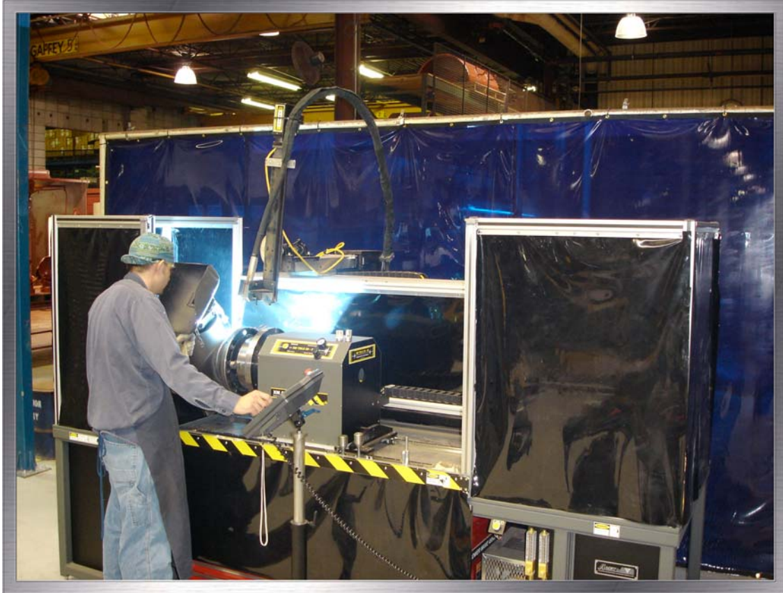
Open-root Pulsed GMAW welding of Carbon Steel Pipe and Forged Flange Components Utilizing Lincoln Pulsed GMAW Waveform Technology with advanced AMET XM Weld Controls
